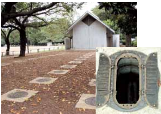
Disaster-ready toilet: Open the manholes shown in the foreground and set up tents over them and they are ready for use as toilets.
