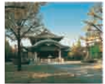
Front of the Tokyo Memorial Hall
